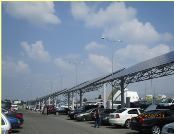
Solar Electricity Generation System
